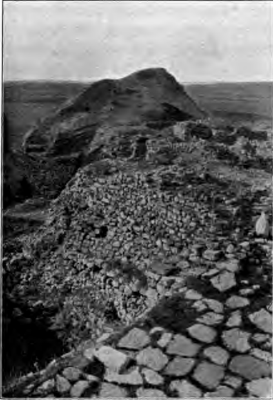
WESTERN WALL OF SECOND STRATUM. Ramp in foreground, Gate FH at back. From N. W. corner of VI. M.
